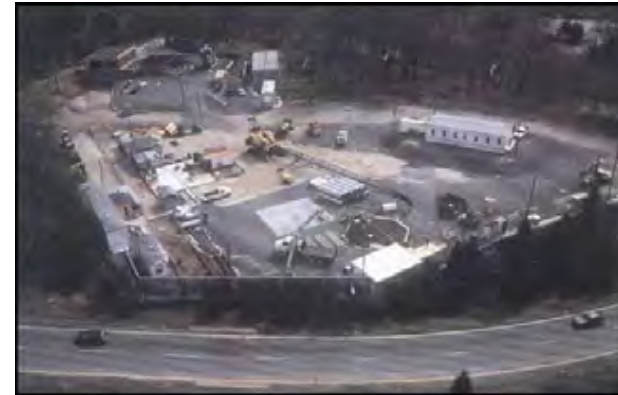
Shaft Site During Construction
