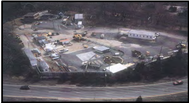
MWWST Shaft 5A with Highway Access
