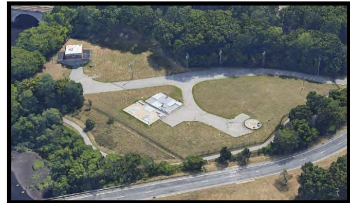
Shaft Site After Construction
